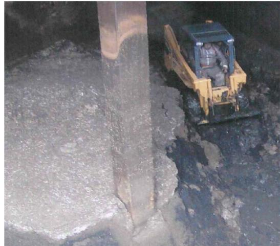
Fig. 3: Labour-intensive removal of sedimented snail shells from an aeration tank
